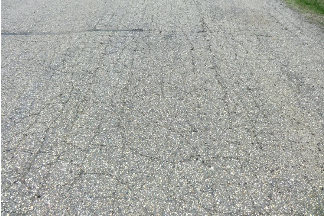
CNB TLA 001 (Alligator Cracking)
